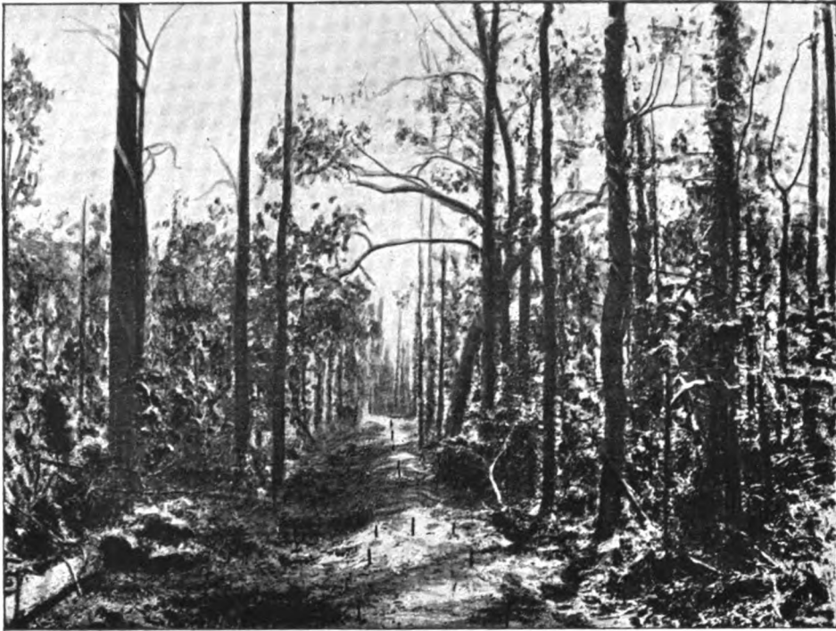
SECTION READY FOR LAYING TRAMWAY.
